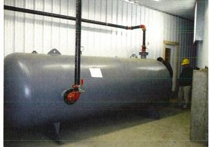
2,120 gallon air receiver (compressed air storage tank)
